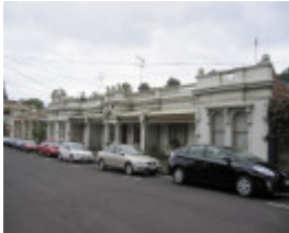
1-11A Shields Street.JPG
