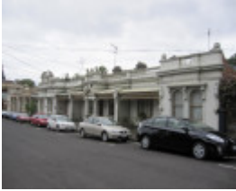
1-11A Shields Street.JPG
