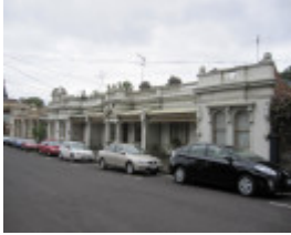
1-11A Shields Street.JPG
