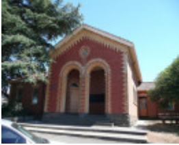
ARARAT COURT HOUSE SOHE 2008
