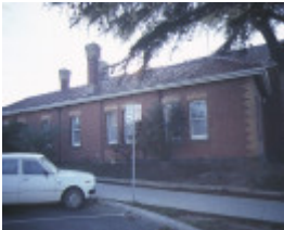
ararat court house side view jun1984
