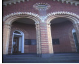
ararat court house entrance detail jun1984
