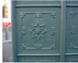
Urinal Nth Melbourne panel detail KJ 21 07 2007
