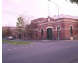
former cable tram engine house rathdowne street carlton north exterior of car shed corner view jun1995
