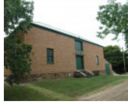
RED BRICK BARN SOHE 2008
