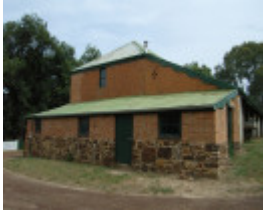
RED BRICK BARN SOHE 2008
