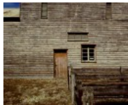
warrock warrock road casterton exterior detail of wool shed publication
