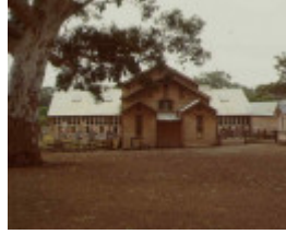
warrock warrock road casterton wool shed front view publication
