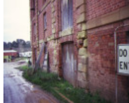
flour mill barker street castlemaine brickwork detail
