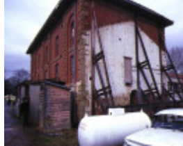
1 flour mill barker street castlemaine front view
