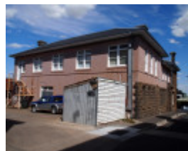
H0618 FORMER ARARAT SUB-TREASURY AND POST OFFICE LHA 2015 3.JPG
