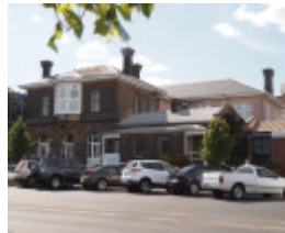
H0618 FORMER ARARAT SUB-TREASURY AND POST OFFICE LHA 2015 1.JPG
