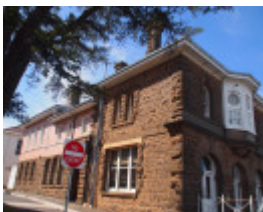
H0618 FORMER ARARAT SUB-TREASURY AND POST OFFICE LHA 2015 2.JPG
