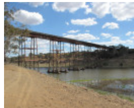
2504_Melton Railway Viaduct_7 November 2009_HV_009_lo res.jpg
