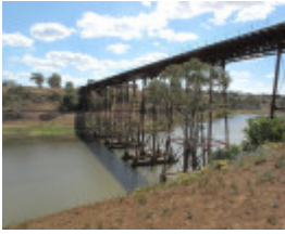
2504_Melton Railway Viaduct_7 November 2009_HV_032_lo res.jpg
