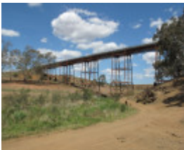
2504_Melton Railway Viaduct_7 November 2009_HV_007_lo res.jpg
