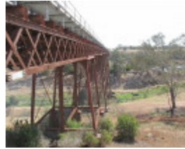
2504_Melton Railway Viaduct_7 November 2009_HV_070_lo res.jpg
