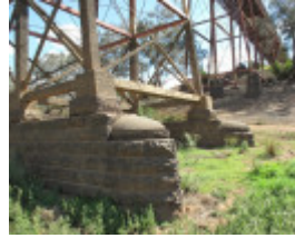
2504_Melton Railway Viaduct_7 November 2009_HV_055_lo res.jpg
