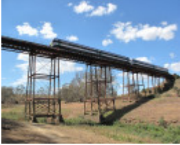
2504_Melton Railway Viaduct_7 November 2009_HV_041_lo res.jpg
