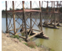
2504_Melton Railway Viaduct_7 November 2009_HV_012_lo res.jpg
