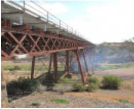
2504_Melton Railway Viaduct_7 November 2009_HV_069_lo res.jpg
