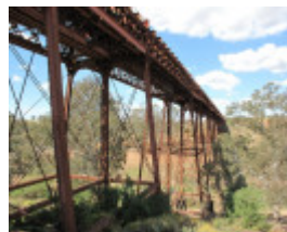
2504_Melton Railway Viaduct_7 November 2009_HV_030_lo res.jpg
