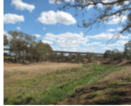
2504_Melton Railway Viaduct_7 November 2009_HV_005_lo res.jpg
