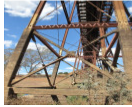
2504_Melton Railway Viaduct_7 November 2009_HV_048_lo res.jpg
