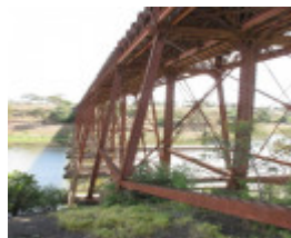
2504_Melton Railway Viaduct_7 November 2009_HV_026_lo res.jpg
