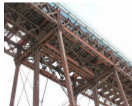
2504_Melton Railway Viaduct_7 November 2009_HV_016_lo res.jpg
