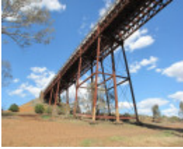
2504_Melton Railway Viaduct_7 November 2009_HV_058_lo res.jpg
