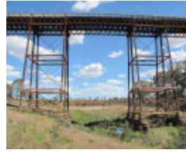
2504_Melton Railway Viaduct_7 November 2009_HV_056_lo res.jpg
