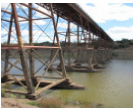
2504_Melton Railway Viaduct_7 November 2009_HV_013_lo res.jpg
