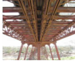
2504_Melton Railway Viaduct_7 November 2009_HV_068_lo res.jpg
