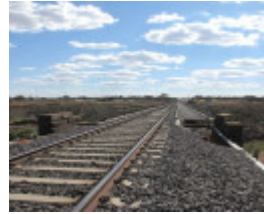
2504_Melton Railway Viaduct_7 November 2009_HV_072_lo res.jpg
