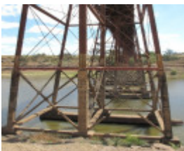
2504_Melton Railway Viaduct_7 November 2009_HV_019_lo res.jpg
