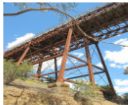
2504_Melton Railway Viaduct_7 November 2009_HV_017_lo res.jpg
