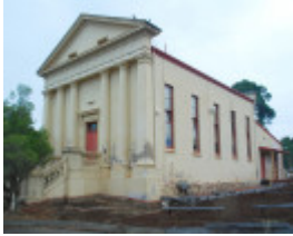
FORMER EAGLEHAWK EAST METHODIST CHURCH SOHE 2008
