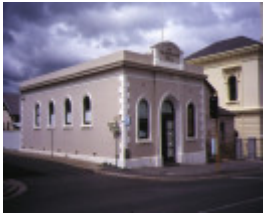
1 former telegraph office & faulder watson hall barker street castlemaine side view faulder watson hall
