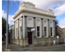
h00580 former state savings bank h0580
