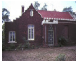
residence farnsworth street castlemaine side view may1984
