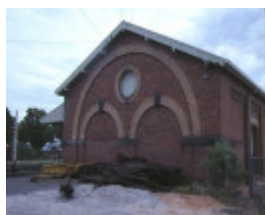
castlemaine railway station complex kennedy street castlemaine railshed end view
