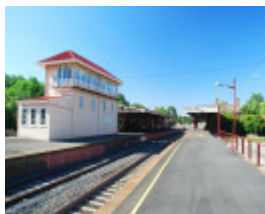
CASTLEMAINE RAILWAY PRECINCT (MURRAY VALLEY RLWY, MELBOURNE TO ECHUCA) SOHE 2008
