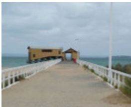
QUEENSLIFF PIER AND LIFEBOAT COMPLEX SOHE 2008
