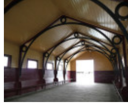
QUEENSLIFF PIER AND LIFEBOAT COMPLEX SOHE 2008
