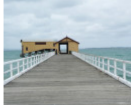
QUEENSLIFF PIER AND LIFEBOAT COMPLEX SOHE 2008
