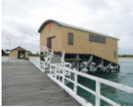
QUEENSLIFF PIER AND LIFEBOAT COMPLEX SOHE 2008
