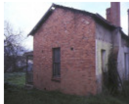
former castlemaine court house goldsmith crescent castlemaine side view
