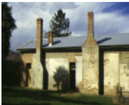
former castlemaine court house goldsmith crescent castlemaine rear view
