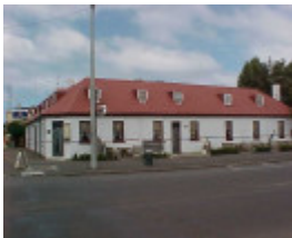
caledonian hotel bank street port fairy side view nov1999
