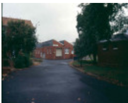
Royal Park Hospital Demolished April 2002
