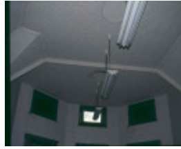
Royal Park Hospital Ward Ceiling April 2002
