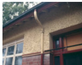
Royal Park Hospital Detail April 2002
