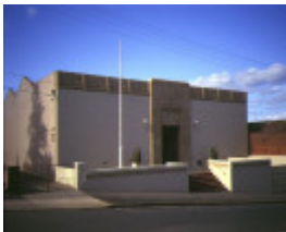
castlemaine art gallery & historic museum lyttleton street castlemaine front facade nov1990
