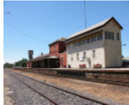
Wangaratta RWS Signal Box & Station Building February 2002
