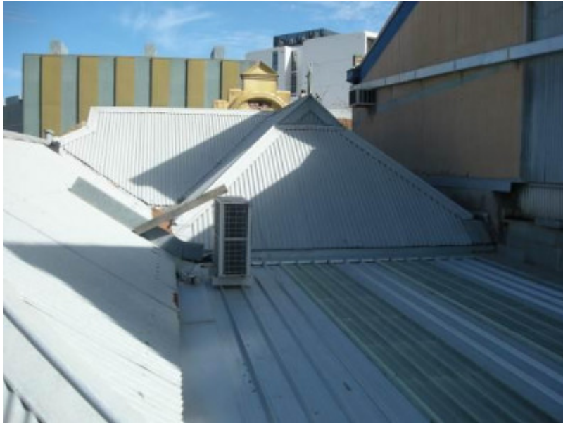
Looking towards the west (Selwyn Street) at the 1896 building's roofscape
