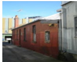
South elevation looking west towards Selwyn Street from un-named laneway
