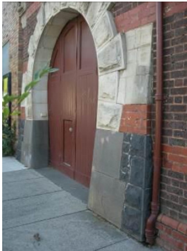
The horseshoe arch integrates limestone, trachyte and basalt with the brickwork
