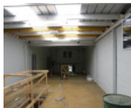
Looking west towards the fire engine room from the space formed by the mid-1950s roofing of the former yard
