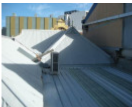
Looking towards the west (Selwyn Street) at the 1896 building's roofscape
