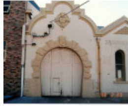
1990: at time of purchase by ABC, prior to removal of exterior paint
