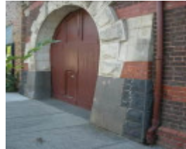
The horseshoe arch integrates limestone, trachyte and basalt with the brickwork
