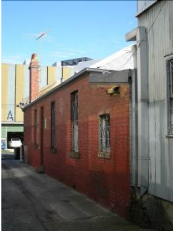
South elevation looking west towards Selwyn Street from un-named laneway
