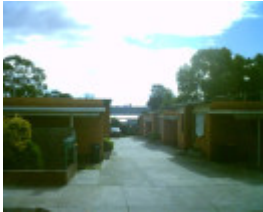
8 William Street (12 Units)
