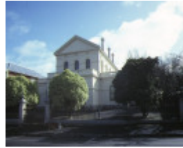
1 castlemaine court house lyttleton street castlemaine front view aug1984
