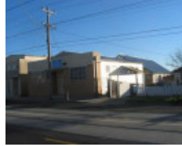
West Preston Progress Hall ii
