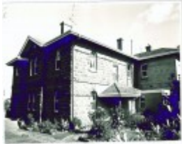
26623 St Ronan's, former Post Office
