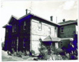
26623 St Ronan's, former Post Office
