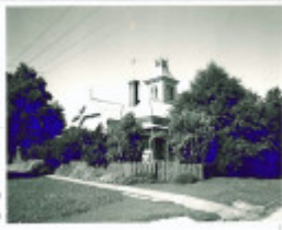
26630 Residence with Tower
