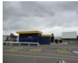
Coburg Drive In_8 May 2009_mz_Projection Building
