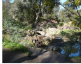
Clifton Bridge, Darebin Parklands, off Separation Street
