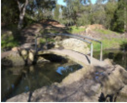
Clifton Bridge, Darebin Parklands (off Separation Street)
