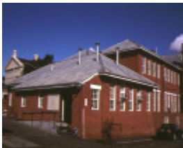
former school of mines lyttleton street castlemaine rear view 1997
