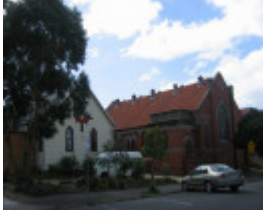
Former Thornbury Presbyterian Church and Hall
