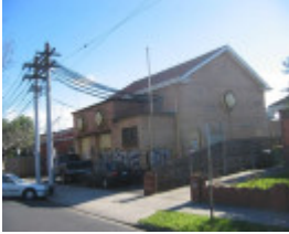
MMTB Substation, 7 Martin Street, Thornbury
