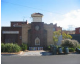
Electricity Substation, Pender Street, Thornbury
