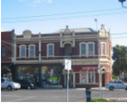
Prince Alfred Hotel (Former) 111-113 High Street
