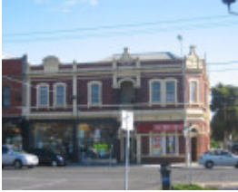
Prince Alfred Hotel (Former) 111-113 High Street
