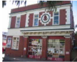
378 High St - Metropolitan Fire Brigade
