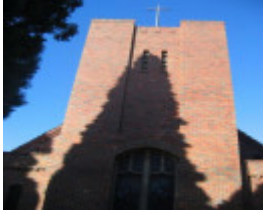
All Saints Anglican Complex, 400 High Street
