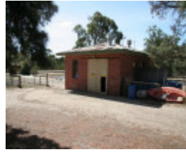
H2167 Lady Northcote Camp Maintenance Shed
