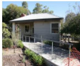
H2167 Lady Northcote Camp Office former Cook's Cottage
