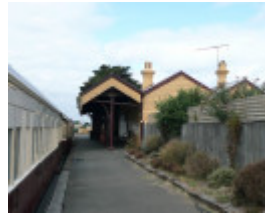
QUEENSCLIFF RAILWAY STATION SOHE 2008
