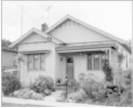
26985 Francis Street No 99 Photo
