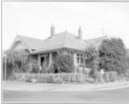
27084 Perth Street No 10 Photo
