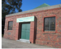
Regent Baptist Church, 726 - 734 High Street, Reservoir
