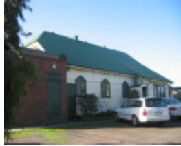
Regent Baptist Church, 726 - 734 High Street, Reservoir
