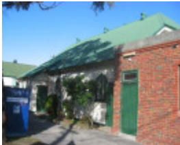
Regent Baptist Church, 726 - 734 High Street, Reservoir
