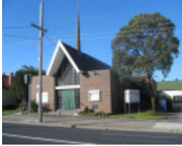
Regent Baptist Church, 726 - 734 High Street, Reservoir
