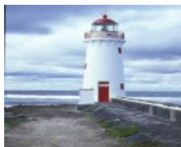
1 griffith island lighthouse griffith island port fairy front view
