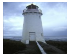
griffith island lighthouse griffith island port fairy rear view
