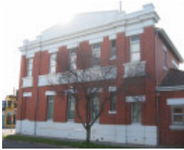
State Savings Bank (Former) 600-606 Plenty Road
