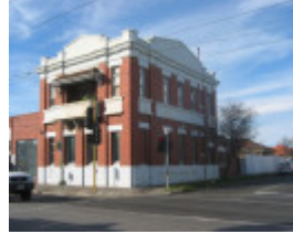
State Saving Bank (Former), 600-606 Plenty Road, Image 2
