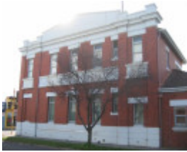
State Savings Bank (Former) 600-606 Plenty Road
