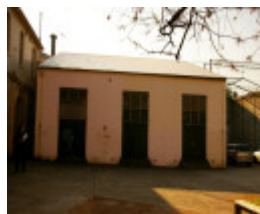
H2170 St Vincent de Paul Boys Orphanage 1958 gymnasium
