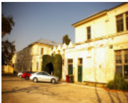
H2170 St Vincent de Paul Boys Orphanage rear Cecil St buildings inc grotto detention plate
