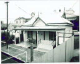
27233 Bowling Club Rooms
