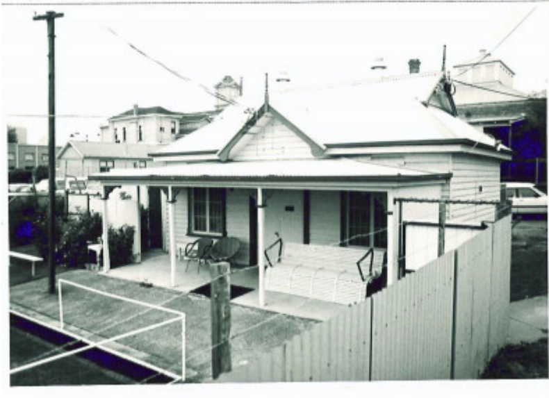
27233 Bowling Club Rooms
