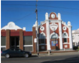
Salvation Army Hall, 710 High Street, Thornbury
