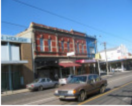
Shop Row 804-810 High Street
