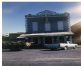
1 former shop & residence templeton street castlemaine front view
