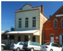
FORMER SHOP AND RESIDENCE SOHE 2008
