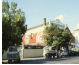
former shop & residence templeton street castlemaine side view
