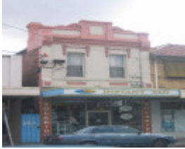
Shop, 283 High Street, Preston
