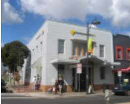
Commonwealth Bank 374-76 High Street
