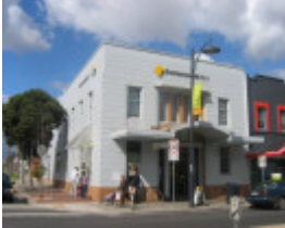
Commonwealth Bank 374-76 High Street
