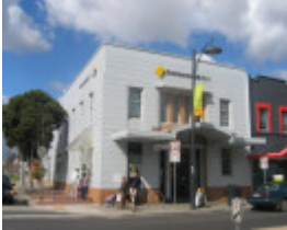
Commonwealth Bank 374-76 High Street
