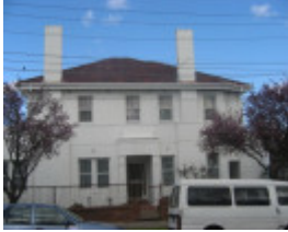
662 High Street, Reservoir
